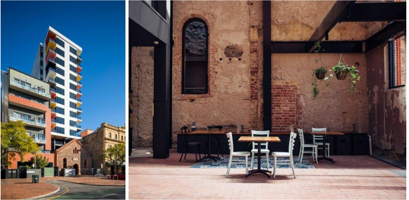
Spence on Light by Tectvs with Mulloway Studio and Hosking Willis Architecture. Photos: David Sievers and Little Mission Cafe
