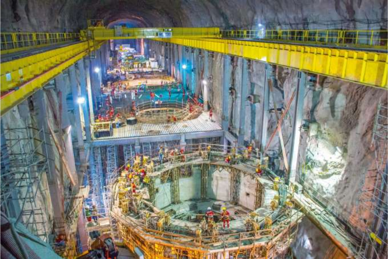
Site works machine hall HPP Laúca, Angola
